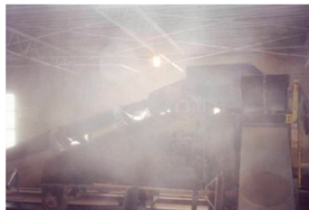
Typical Class II Dust Location
